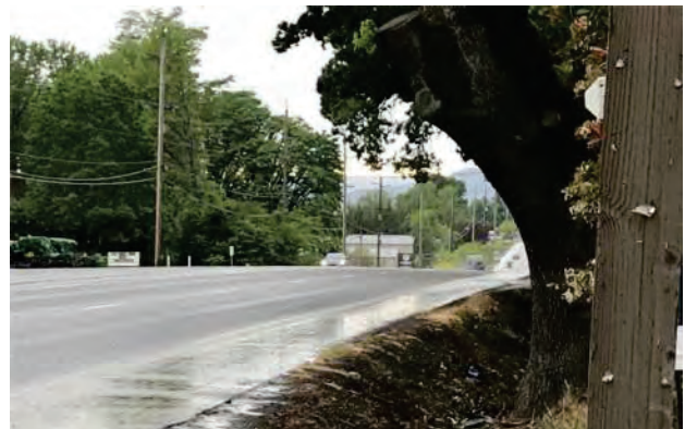
At 336 th Avenue looking west
