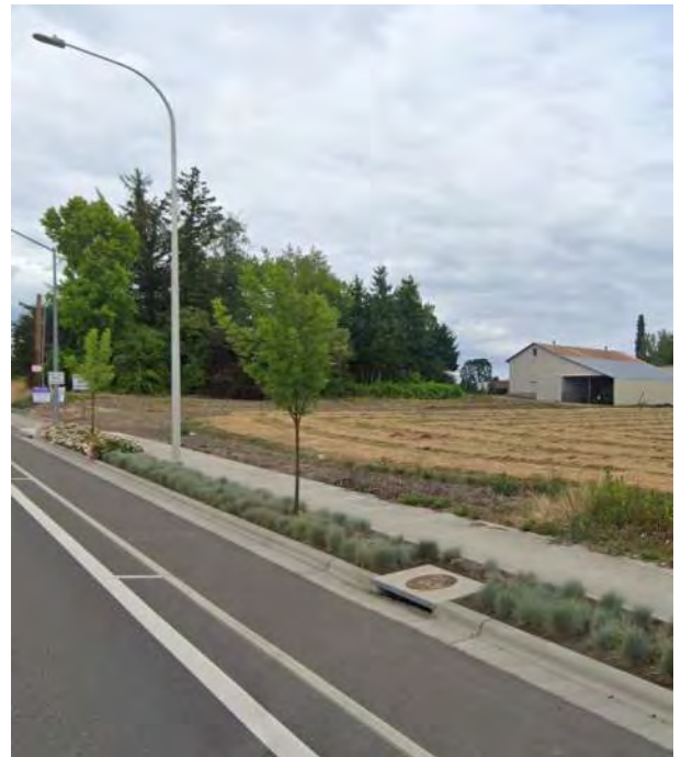
Example of separated pedestrian facilities on Brookwood Parkway in Washington County, OR
