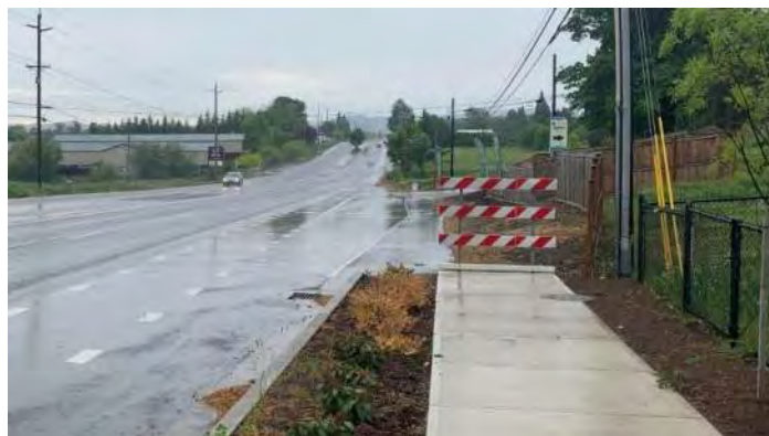
Examples of locations on OR 8 where sidewalk ends abruptly under current conditions
