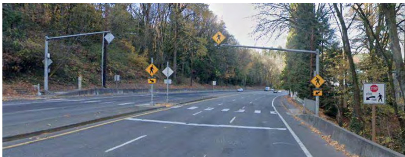
Example of Overhead RRFB Installation
