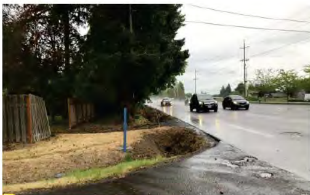
At 336 th Avenue looking east
