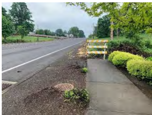
Examples of locations on OR 8 where sidewalk ends abruptly under current conditions
