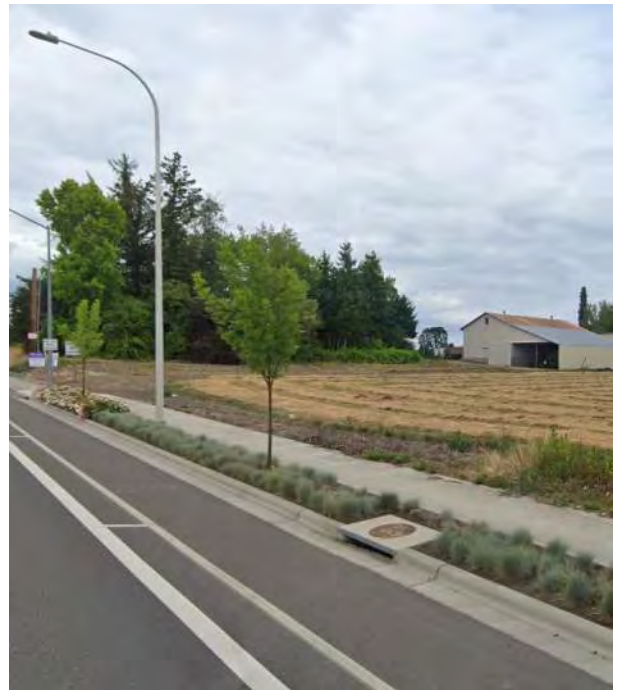
Example of separated pedestrian facilities on Brookwood Parkway in Washington County, OR
