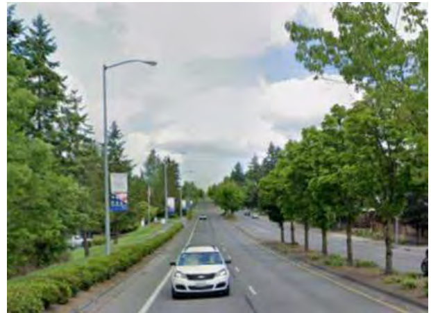
Typical roadway lighting along a multilane facility
