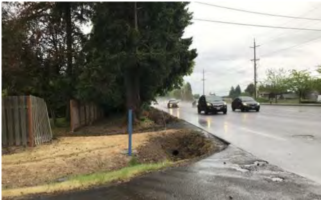
At 336 th Avenue looking east
