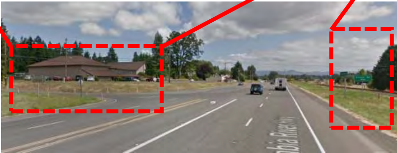
Example of delineators and additional street name signs to increase intersection visibility on Highway 30 Source: Google Streetview
