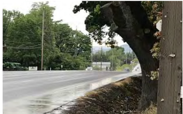
At 336 th Avenue looking west
