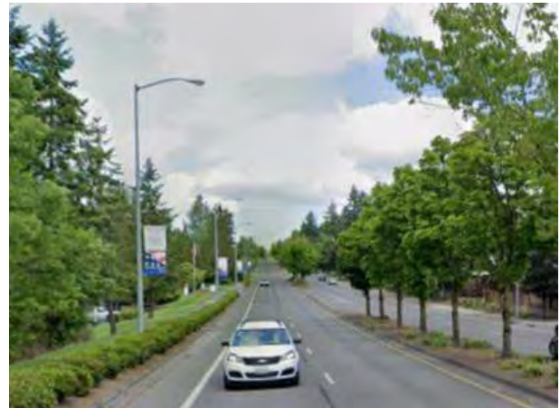
Typical roadway lighting along a multilane facility
