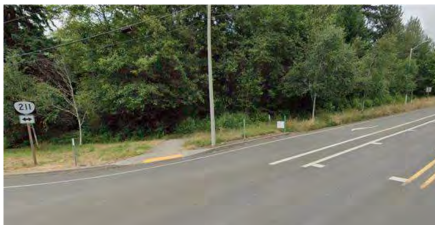
Example in-lane lateral striping installation, OR 211 south of Sandy Source: Google Earth
