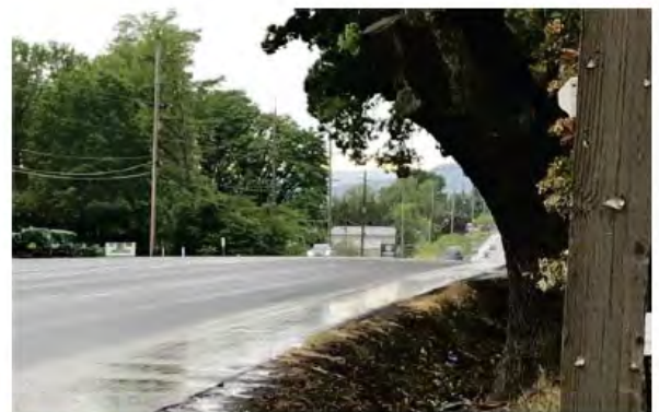
At 336 th Avenue looking west
