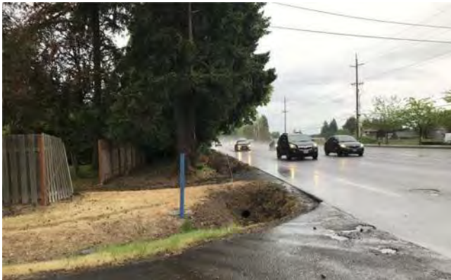
At 336 th Avenue looking east
