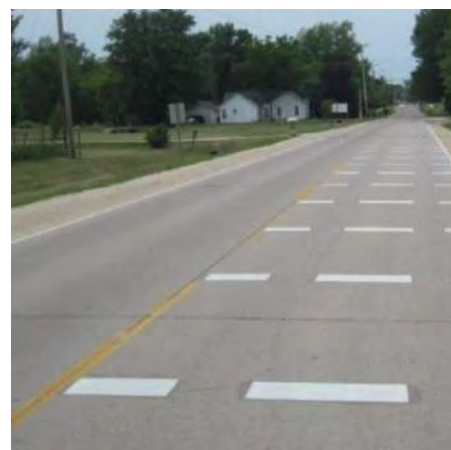
Optical Speed Bars Source: FHWA
