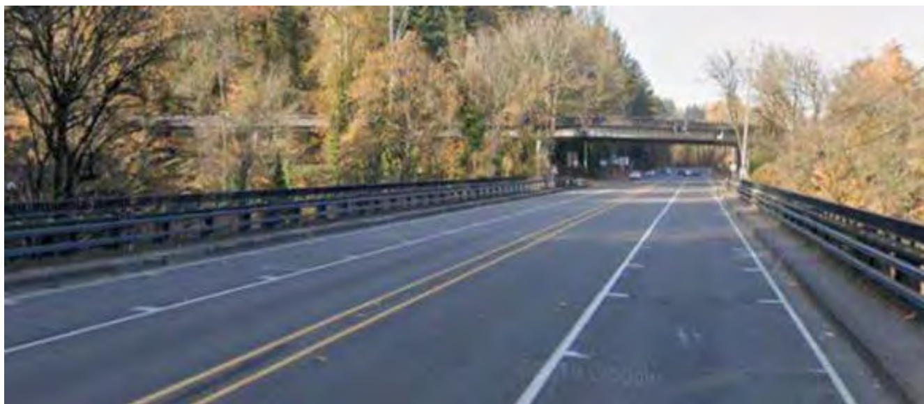
Example installation of in-lane lateral striping on Barbur Boulevard south of Sandy
