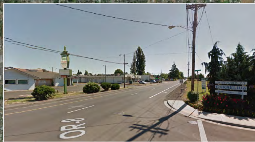
5.5 acres of greenfield and redevelopment opportunity at western Cornelius gateway at OR 8
