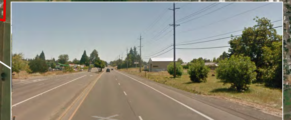
Major stretches of OR 8 within City lacking frontage improvements or productive development
