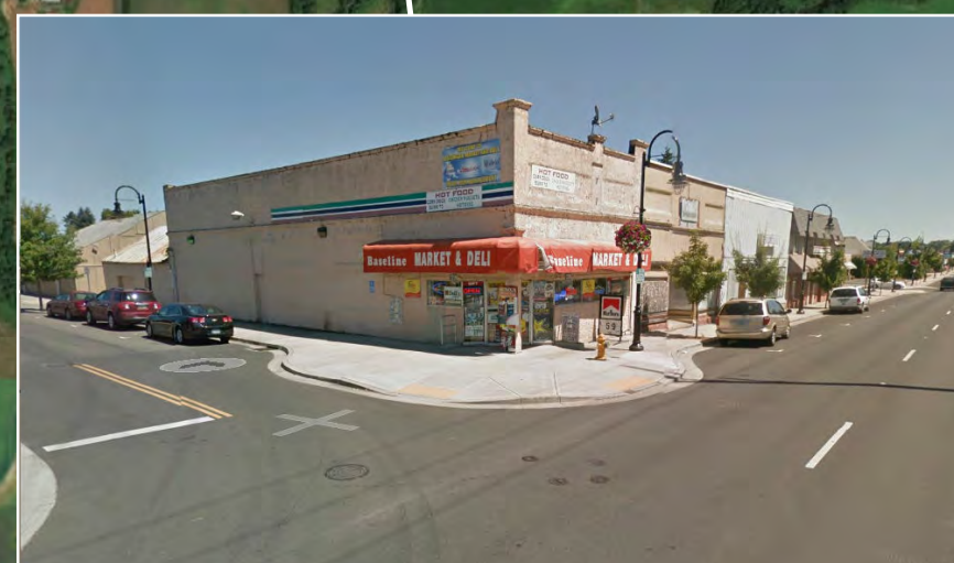
Sorely dilapidated downtown buildings, paired with new pedestrian amenities
