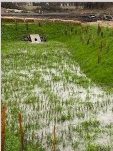
Laurel Woods Water Quality Facility
