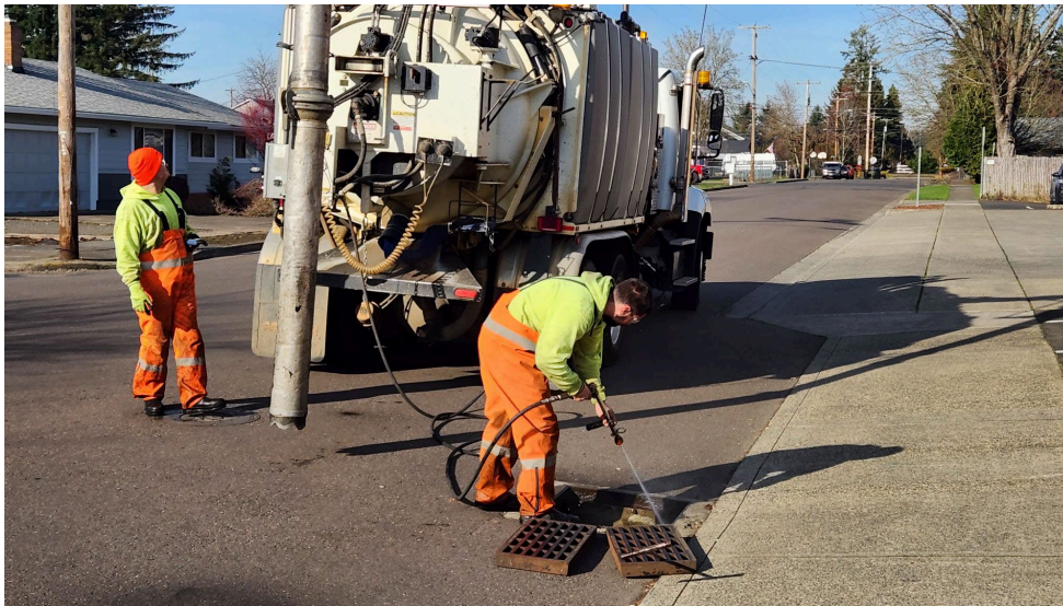
Staff cleaning a Storm Drain
