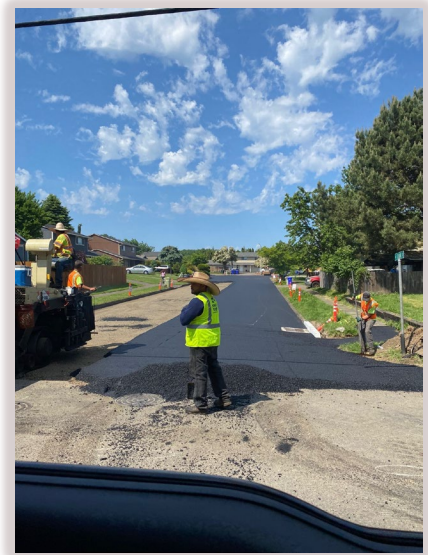
Repaving North Clark Street
