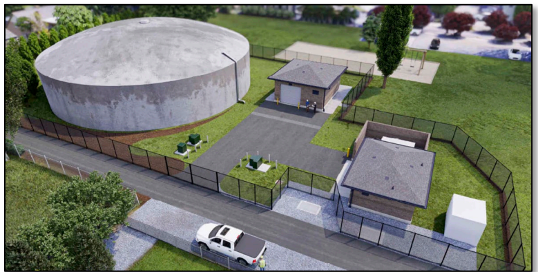
Existing reservoir (left), new Booster Station (center), and ASR facility (right)
