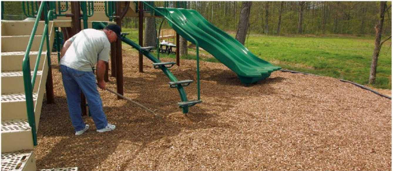
Raking loose-fill engineered wood fiber material
