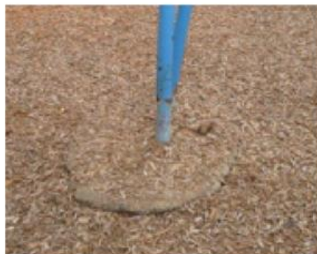
Exposed concrete footing (others)
